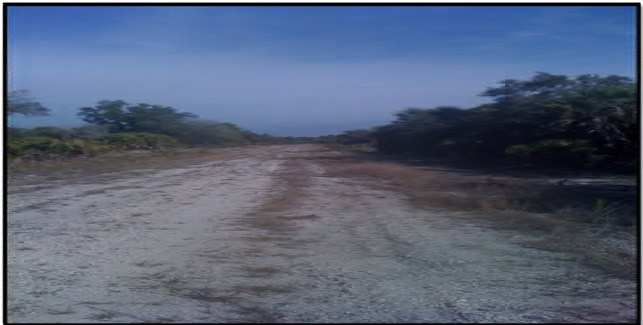
Figure 2.3: Photograph of existing roadway; facing north.
