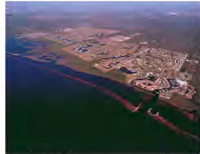
Burnt Store Aerial
